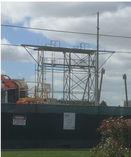
King Street structure soon to be removed
