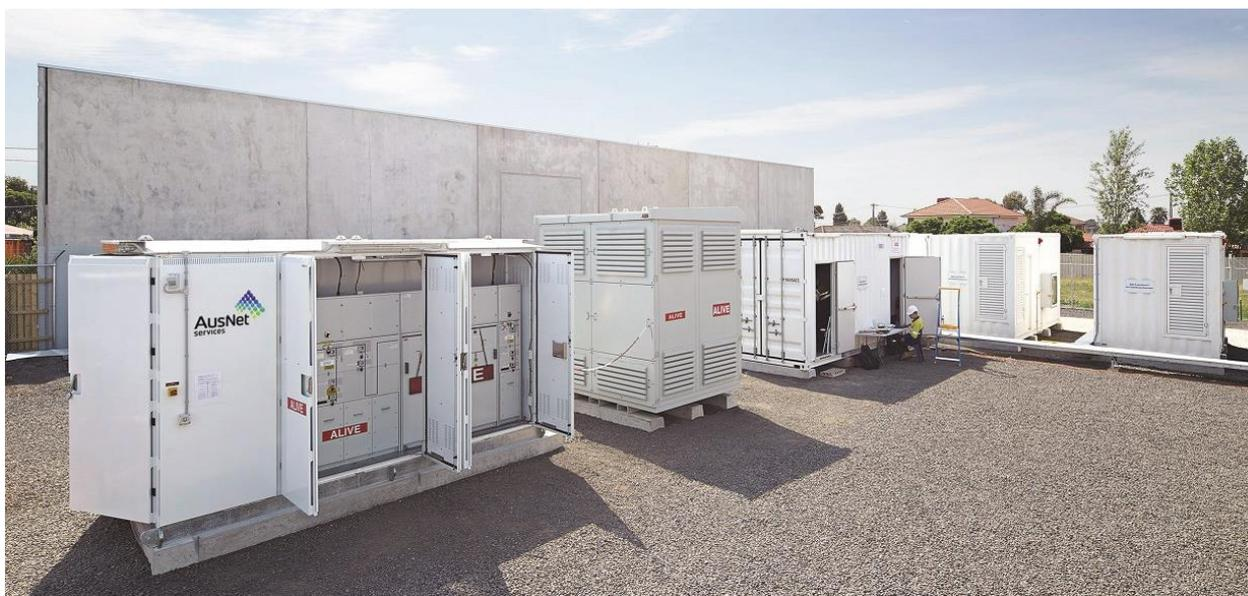
Fig 1: The AusNet Services Grid Energy Storage System, installed in Thomastown (Photo credit: ABB)
