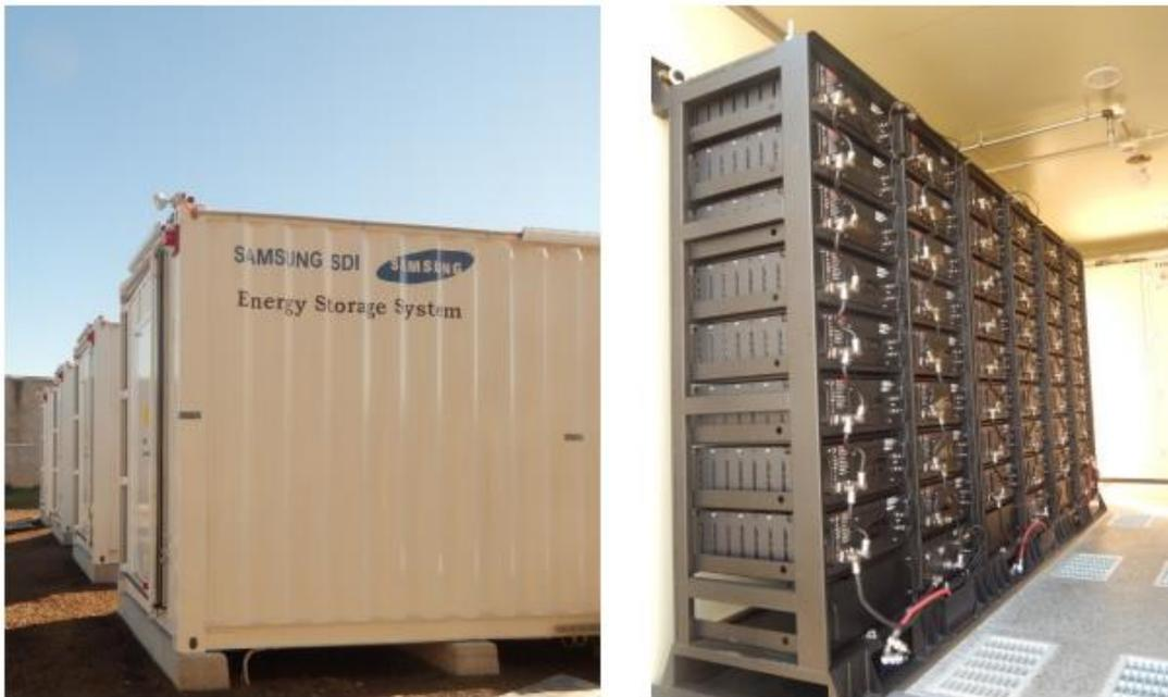
Fig 3 Samsung battery container (left) and battery racks (right)
